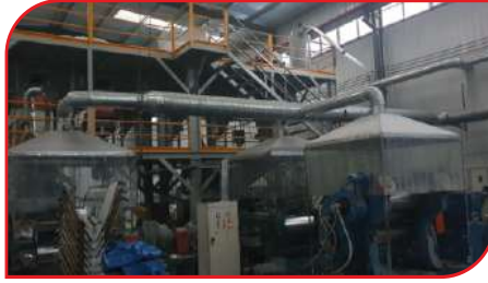
LARGEST IN HOUSE RUBBER MIXING FACILITY
